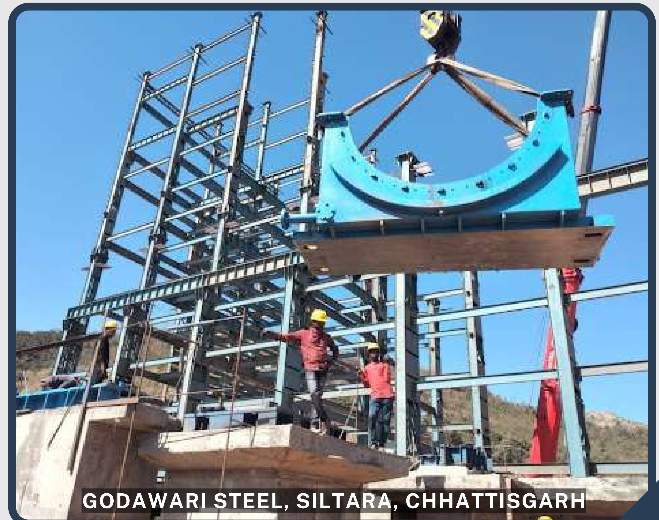
CHIMNEY ERECTION 100 MTR AT UNIT-2
